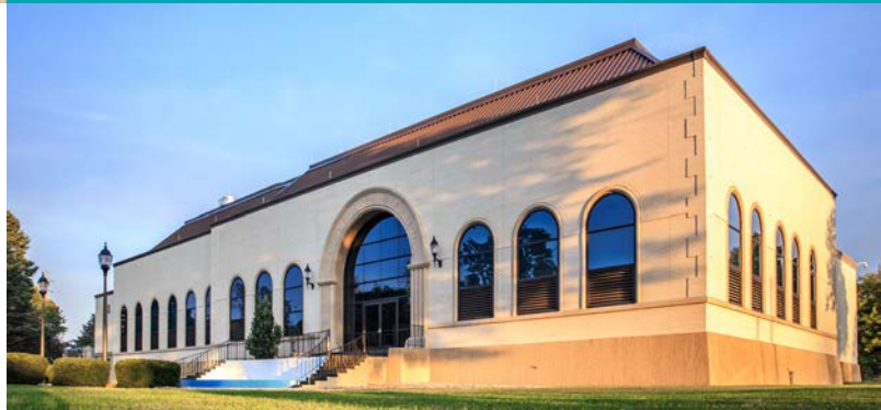
Florence Water Treatment Plant
